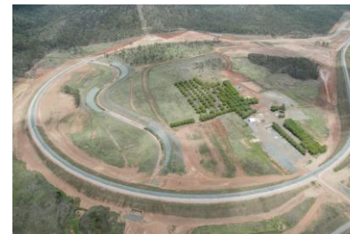
Wiggins Island Rail Loop
